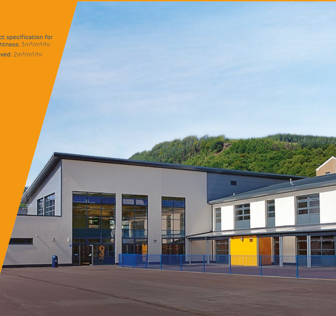
Abercynon Primary School, South Wales
