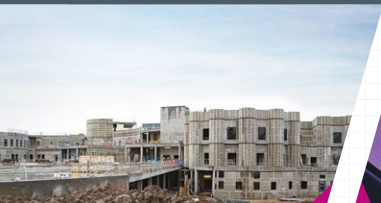
Northumbria Specialist Emergency Care Hospital
